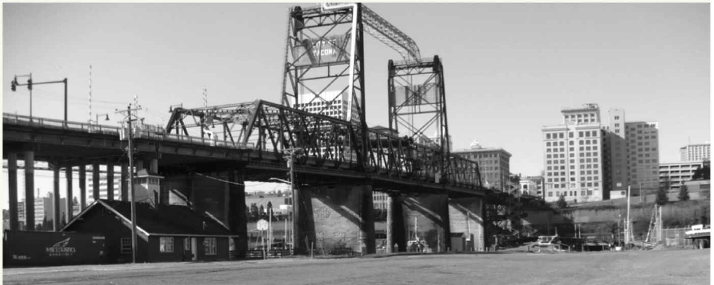
A VIEW OF THE MURRAY MORGAN BRIDGE, GATEWAY TO THE EAST THEA FOSS AND PORT FROM DOWNTOWN TACOMA CREDIT CHARIS HNIN
