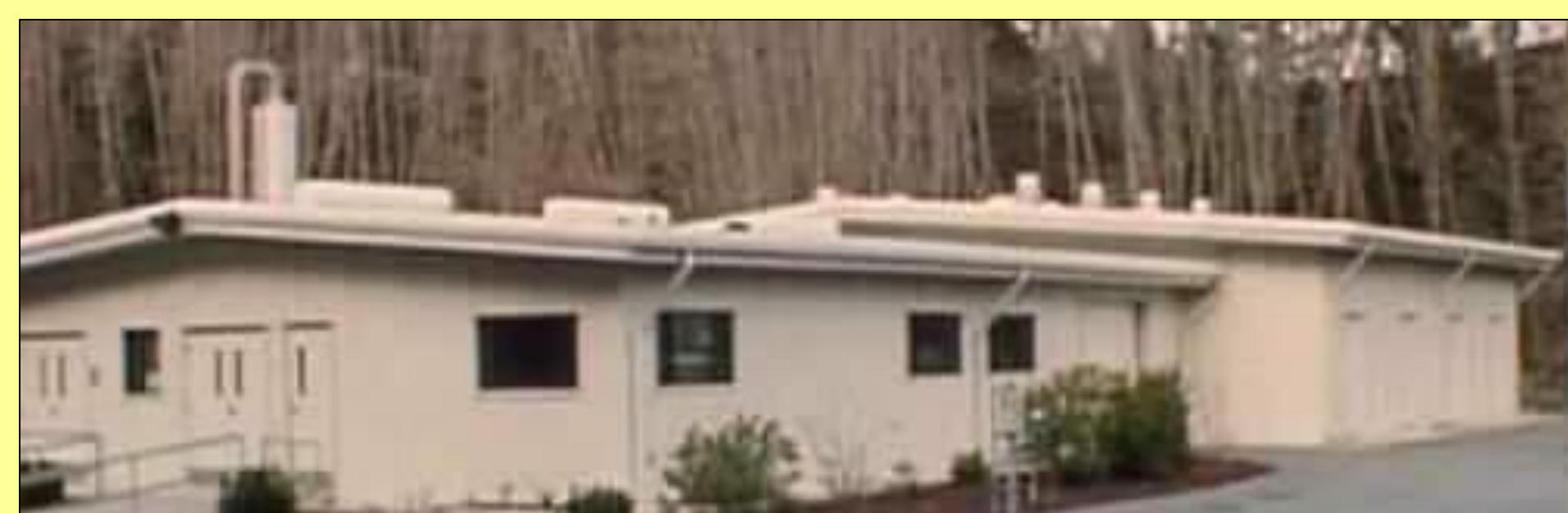
Main building Minter Creek Salmon Hatchery.
