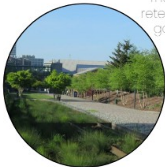
"The Prairie Line Trail bio-retention facility (aka "rain garden") treats runoff from 42 acres" © Images courtesy of 2024 University of Washington Tacoma
