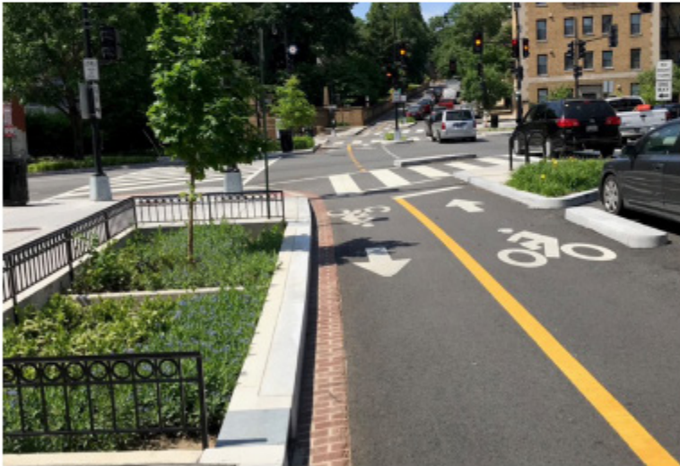
A "green street" uses practices such as porous pavement and bioretention to capture, infiltrate, and evapotranspire stormwater, preventing contaminated runoff from reaching local waterbodies.
