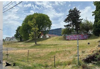
Ginkgo tree and JLS foundation wall. Captured in May 2026 by Nam Cao
